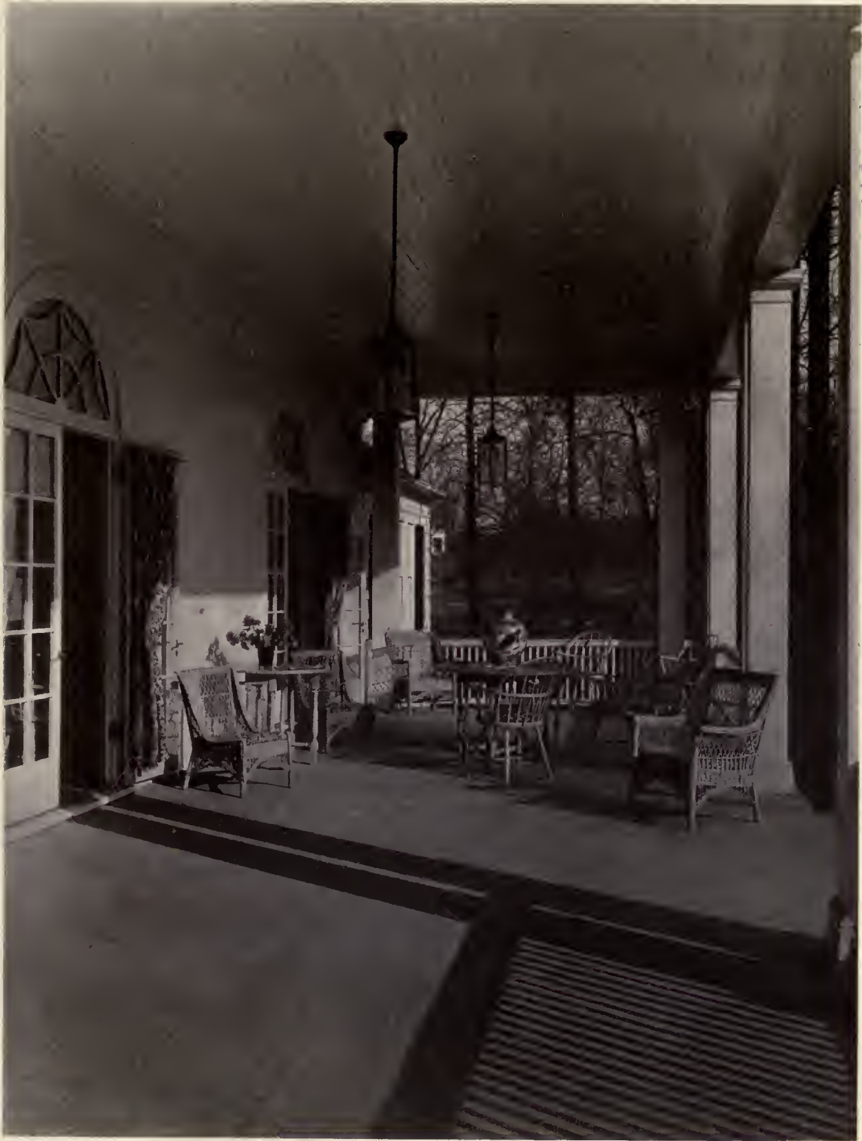
VIEW ON PORCH RIVERDALE COUNTRY CLUB, RIVERDALE, N. Y. DWIGHT JAMES BAUM, ARCHITECT
